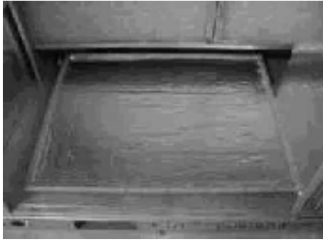
FIGURE 14 - RETURN DOWNFLOW PLENUM WITH PANEL
