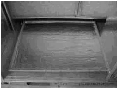
FIGURE 14 - RETURN DOWNFLOW PLENUM WITH PANEL
